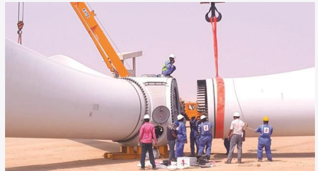
Source: Workers erecting a wind turbine at the Gul Ahmed Wind farm in Pakistan, Private Infrastructure Development Group (PIDG), 2015.
