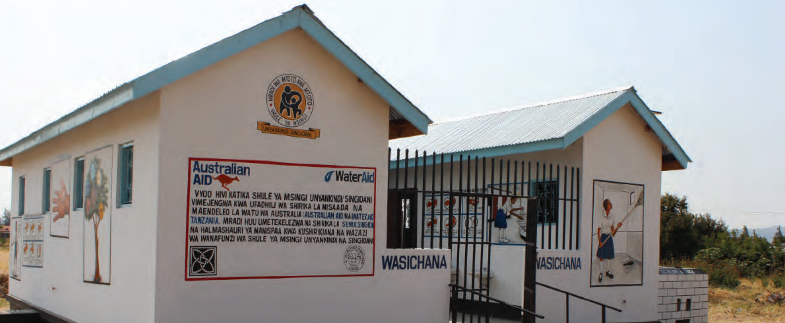
A newly built latrine by WaterAid at Mpalanga Primary School in Dodoma region, Tanzania. 'We were previously embarrassed when using the old toilet block, especially during menses (menstruation), because everyone would know but now no one notices. We no longer have to go home and change, and there is a place to wash ourselves,' says Salvina Maswaga a pupil at Mpalanga. Photo by Douglas Waudo / AACES Resource Facility
