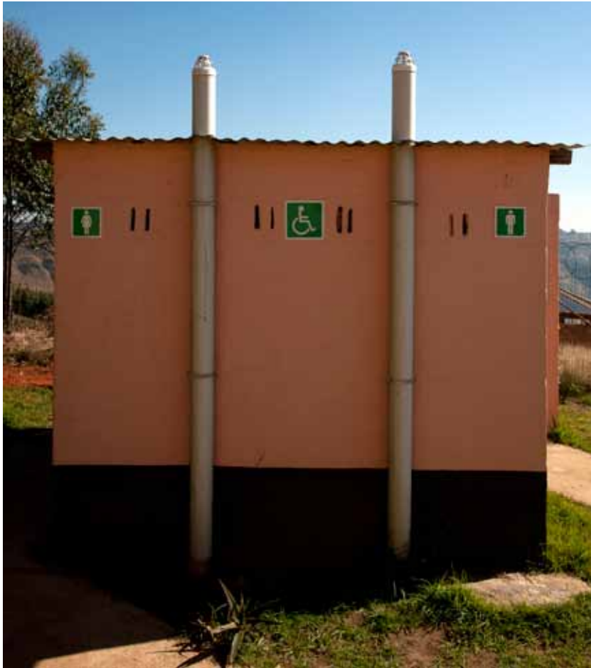
The new toilet at Woza Moya, South Africa for people with disability. Photo by Xavier Vahed. Oxfam, South Africa.
