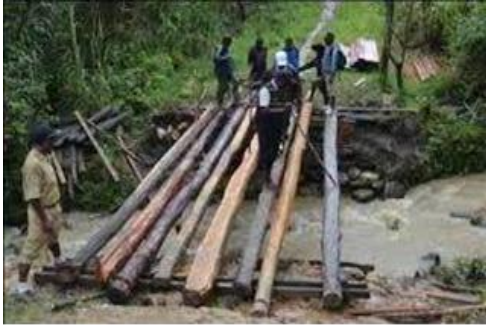
Picture 5.4: Wooden Bridge
