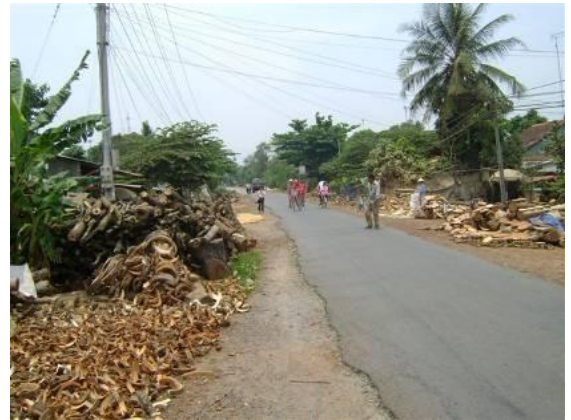
8 - Immediately to the East of the Vam Cong Bridge site on NH54.
