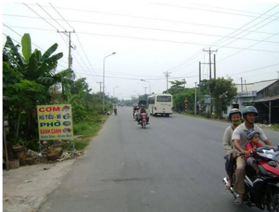
1 - Start of the project looking North along NH-30 – the site of a half-diamond interchange
