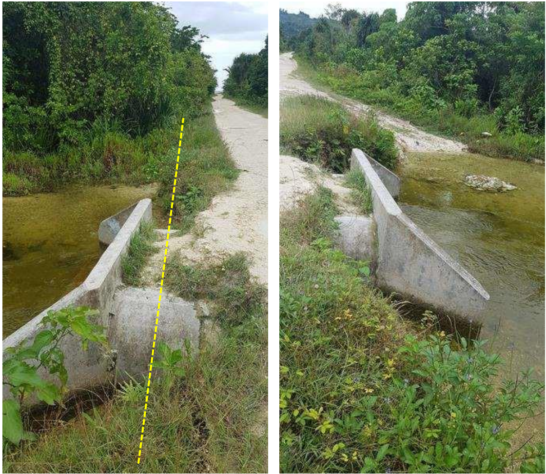
Figure 2-13 Crossing culverts over Langa-linga freshwater lagoon
