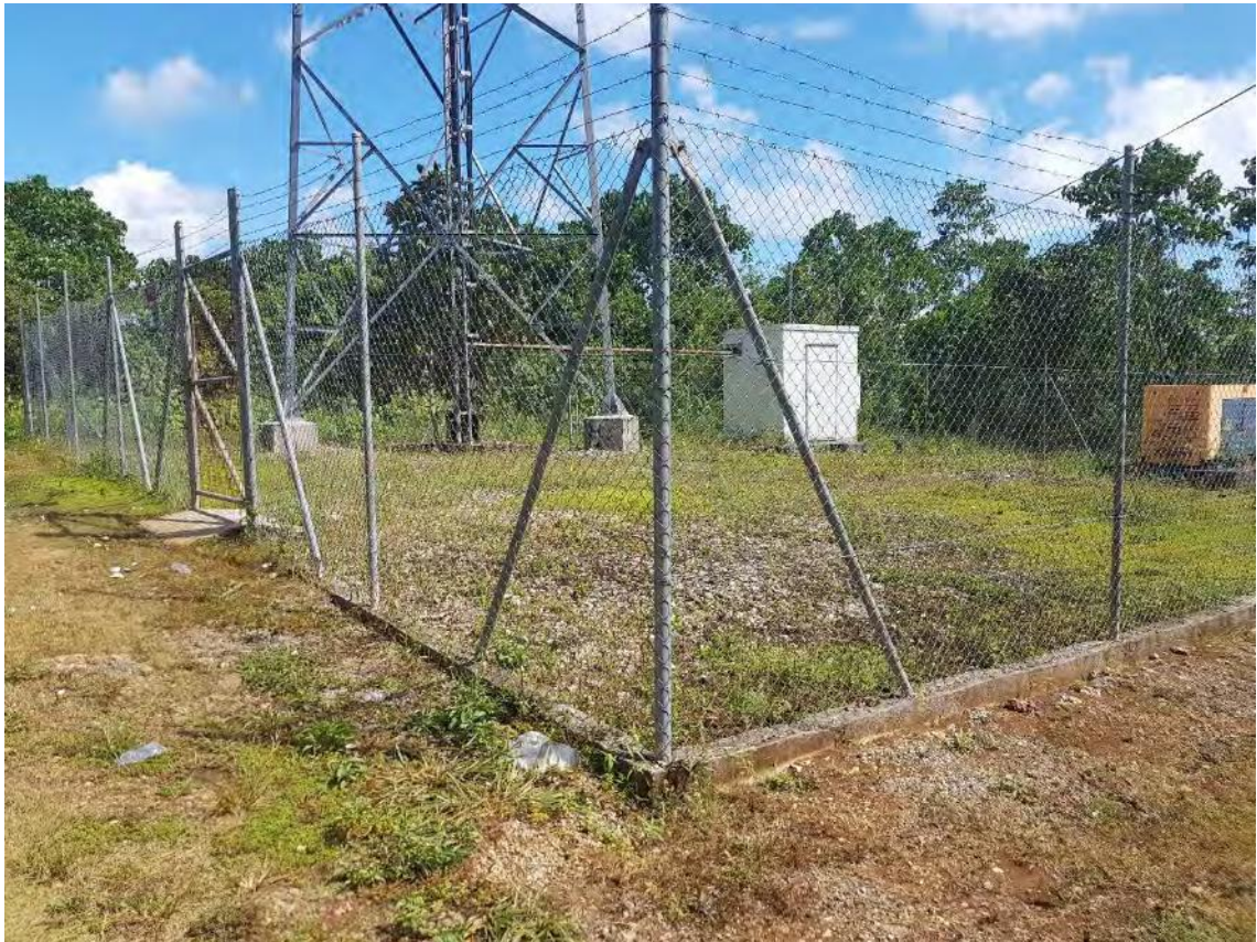
Figure 2-8 View of Telekom compound for the proposed CLS (Vocus, 2018)
