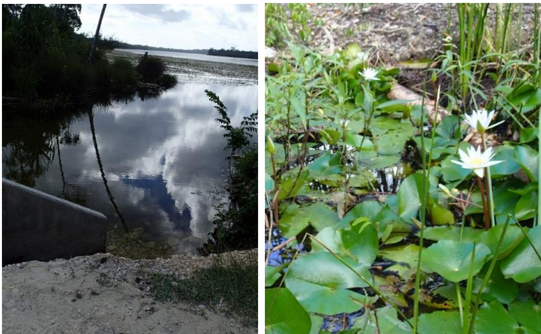
Figure 3-12 Lake (left) showing road edge and culvert; drainage point into lake on right side road (right) showing limited water body
