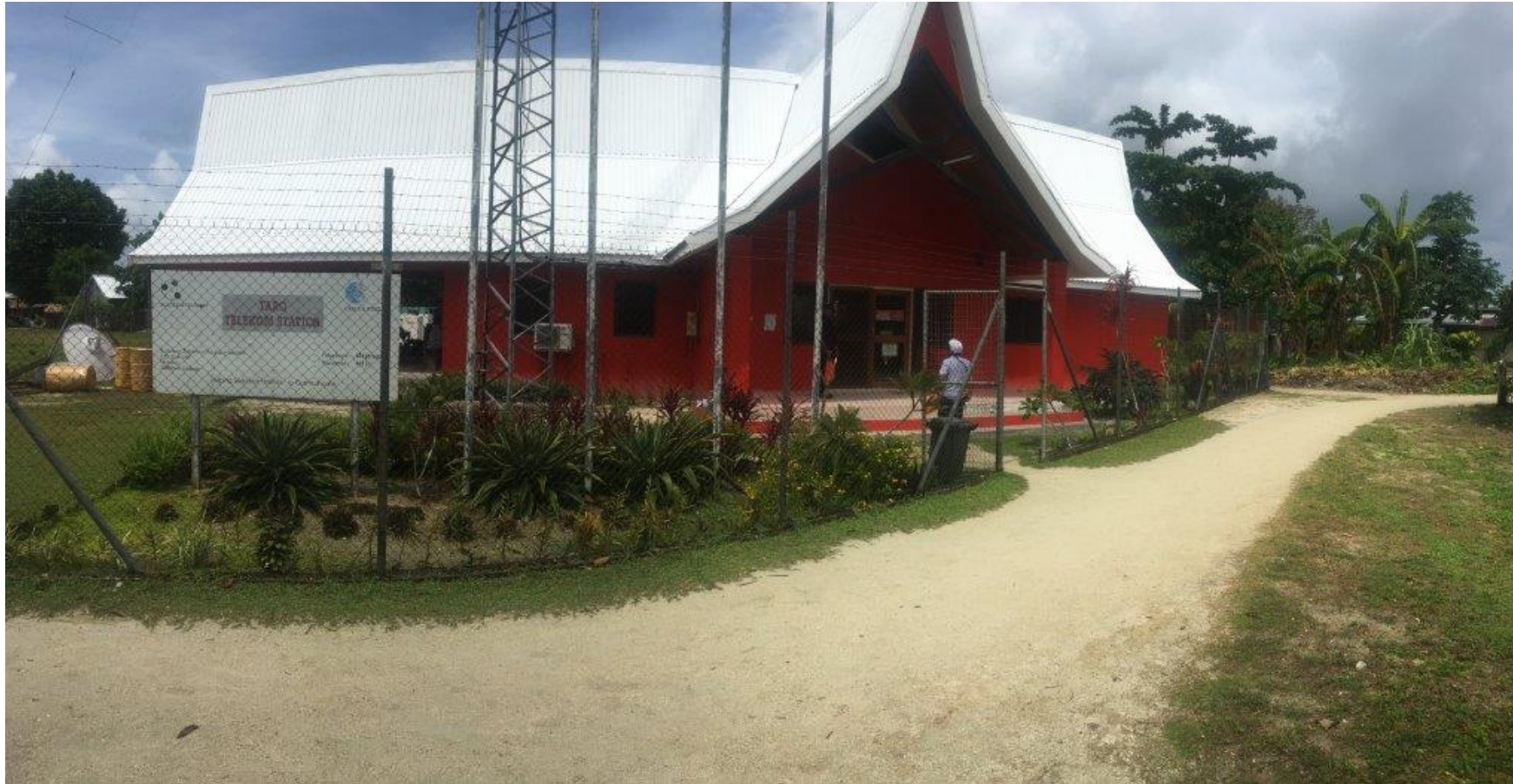
Figure 5-9. Solomon Telekom building immediately landward of one of the proposed landing locations.
