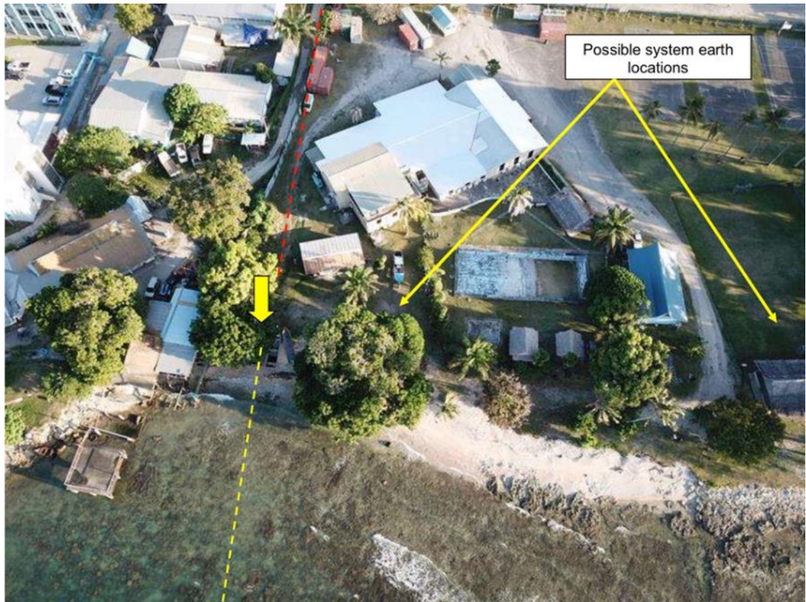
Figure 2-2 Aerial view of Honiara cable landing point and BMH with marine (yellow) and terrestrial (red) routes indicated
