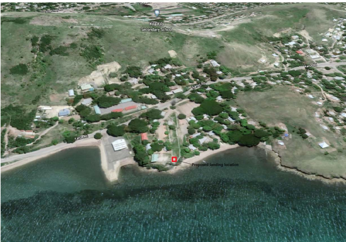
Figure 6-3. Close up of the proposed landing location at Kila Police Barracks.
