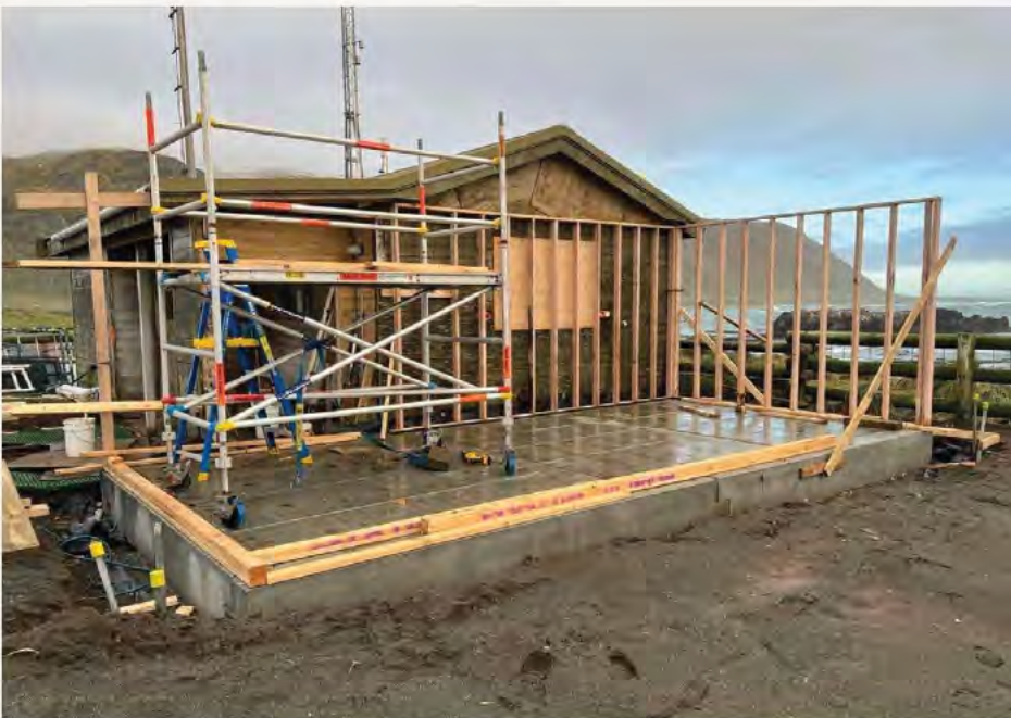
The reconstruction of the Radionuclide Monitoring Station at Macquarie Island, Australia.
