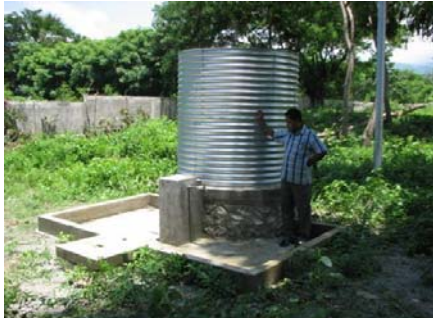
A non-wheelchair accessible tank stand used at a water and sanitation training unit in Tibar.
