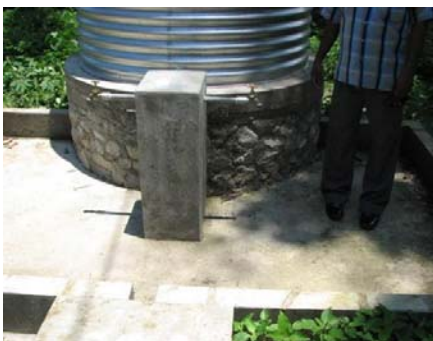
Non-wheelchair accessible taps
