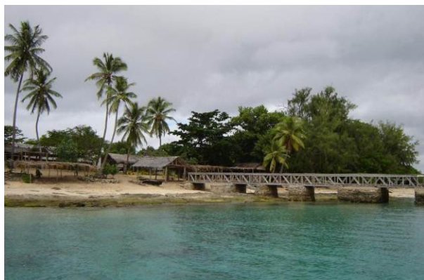
Wharf, Wala Island
