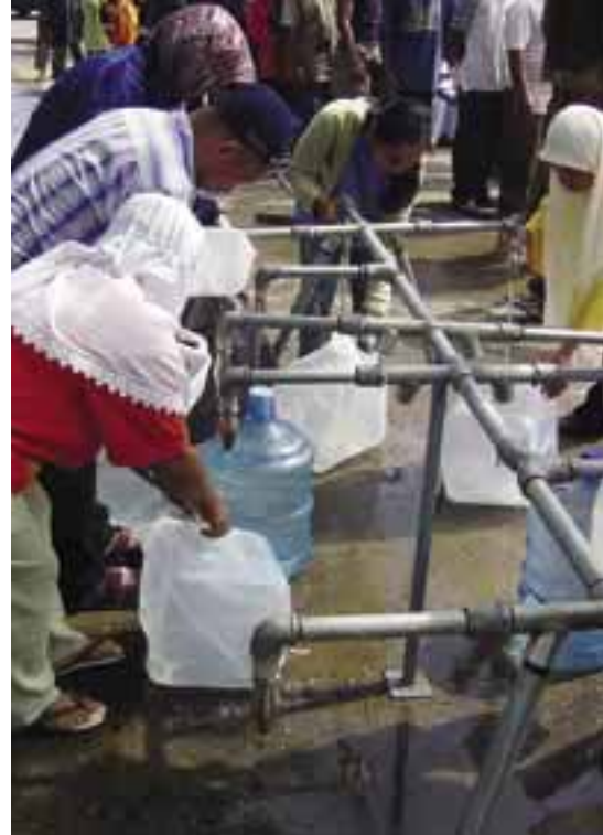
Australian water purification and distribution station, Banda Aceh. In the aftermath of the Indian Ocean tsunami, Australian relief was among the first to arrive in Indonesia. PHOTO: Rob Walker
