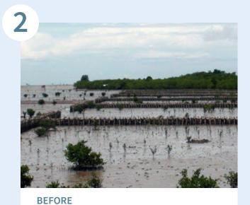
Erosion site with first new sedimentation due to breakwater fences and some planted mangrove seedlings
