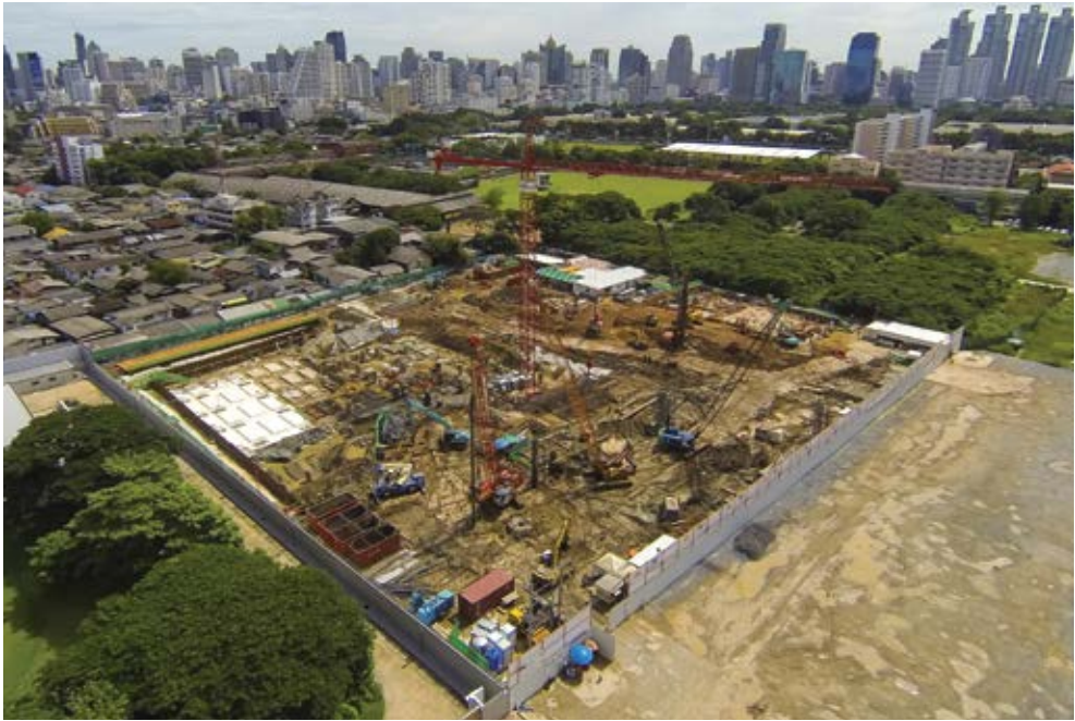
Bangkok embassy complex under construction, 9 September 2014. [DFAT]
