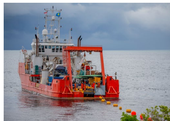
Belau Submarine Cable Company cable laying in Republic of Palau, as part of the AIFFP's Palau Submarine Cable Branch System Project. Credit: Jesse Alpert / Belau Submarine Cable Company
