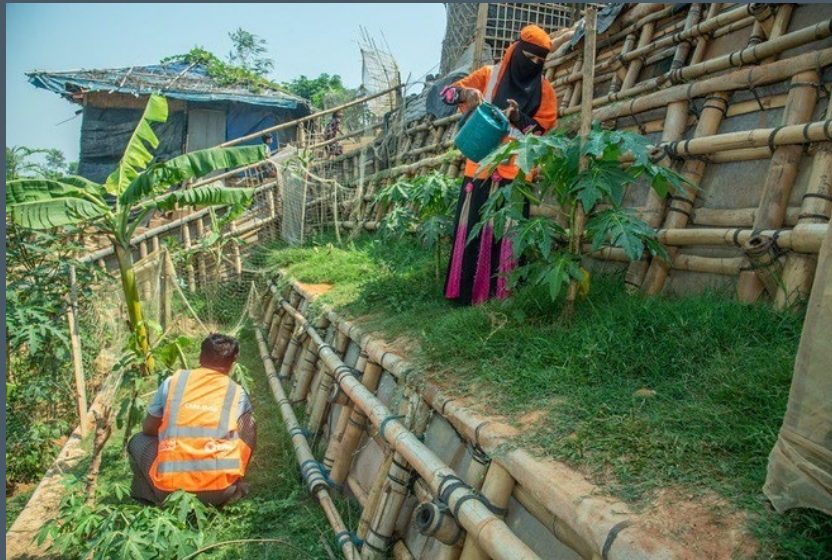
Above: Women and men volunteers worked together to build and grow vegetation on slope stabilisers in refugee camps in Cox's Bazar. Source: Australian Humanitarian Partnership
