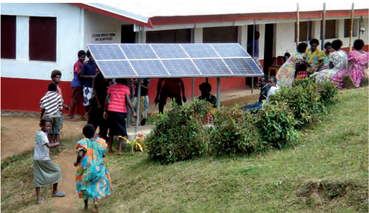
Renewable energy-based systems like this two-kilowatt solar system installed at Coconak Primary School in Vanuatu under a SOPAC project bring electricity and lighting to isolated rural areas. EDD evaluated the implementation of the project.
