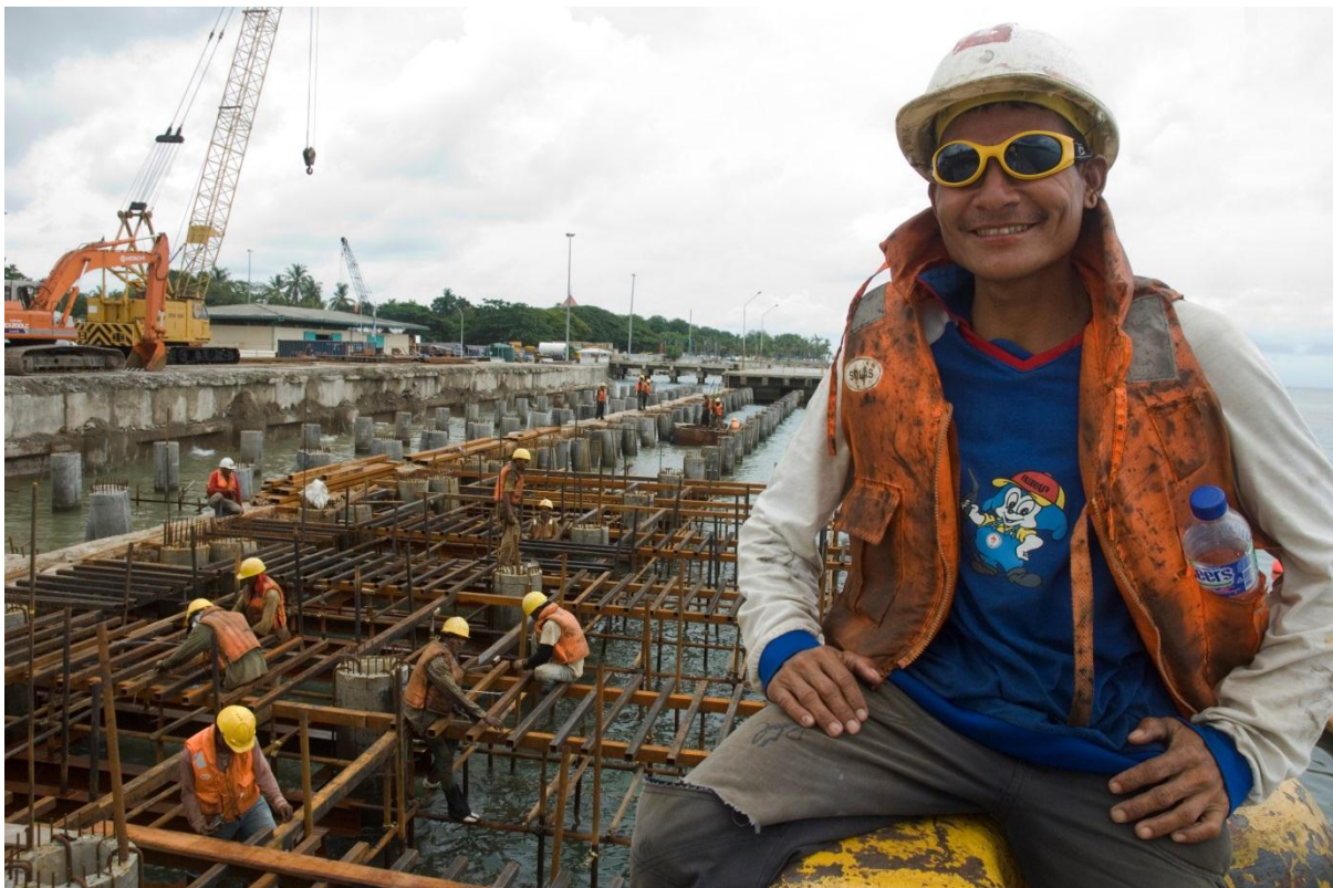
Port construction in Dili, 2008. Photo: Lorrie Graham, AusAID.
