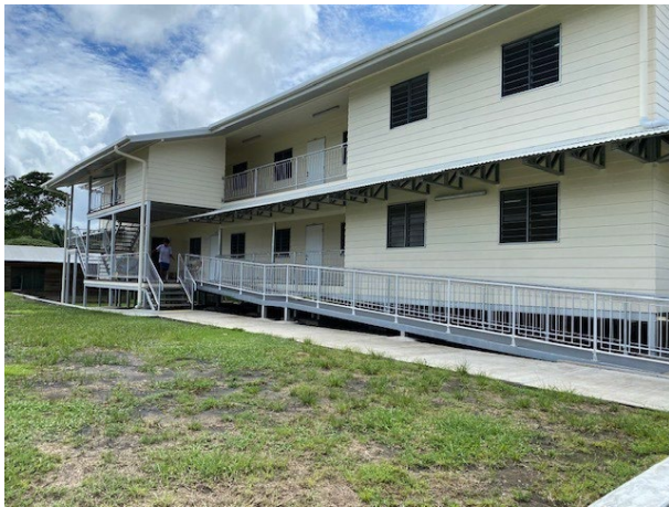
Image above: The Bougainville Technical College has benefited from the construction of new buildings, including the Business Studies building shown here. Even though BTC has no allocated maintenance budget or staff, the building appears to be well-maintained.
