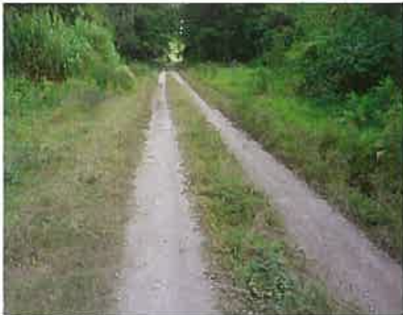
This wheel track road on Tanna provides a comfortable 40 kph ride on a 'non-core' national road – a 'fit-for-purpose' road.
